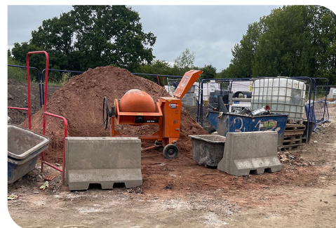
1.2m Concrete Jersey Barriers on site
